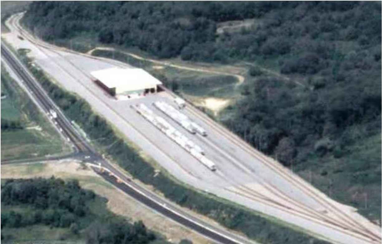
Aerial view of our Ethanol Rail-to-Truck Transloading Terminal in Mt Pleasant, PA
